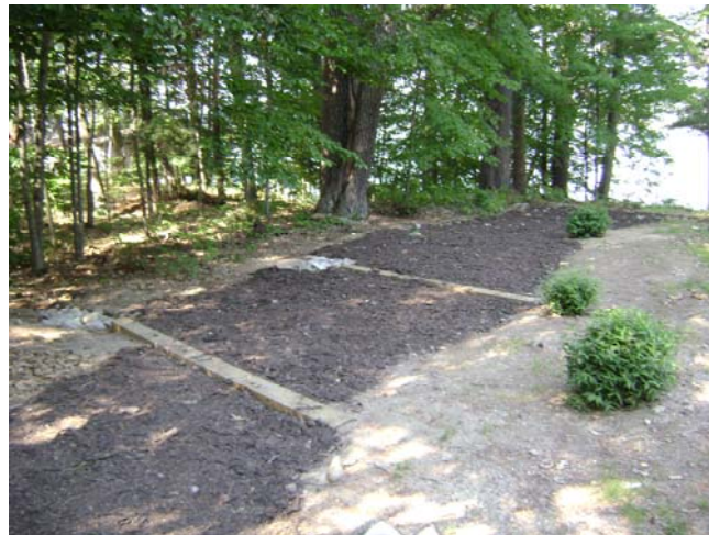
AWWA YCC project on Province Lake - Water bars and Erosion Control Mulch (ECM)
